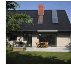
2008-2010 Home Energy, Tilst
