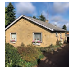
2018-2022 Healthy Homes - Renovation, Randers
