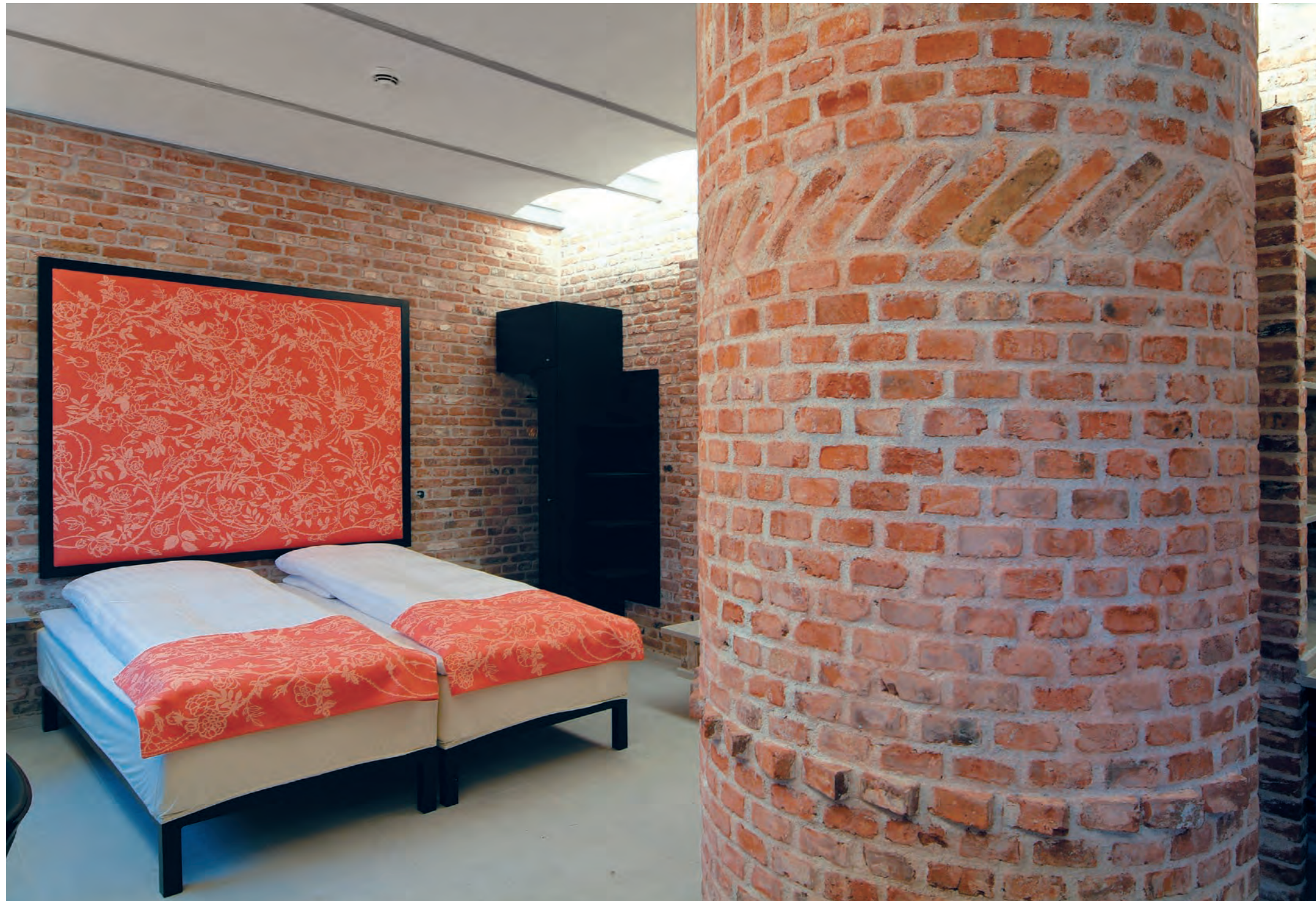
Hotel room in the former farm building at Hindsgavl Castle. The reused bricks are not just aesthetically pleasing, they also reduce the building's carbon footprint.
