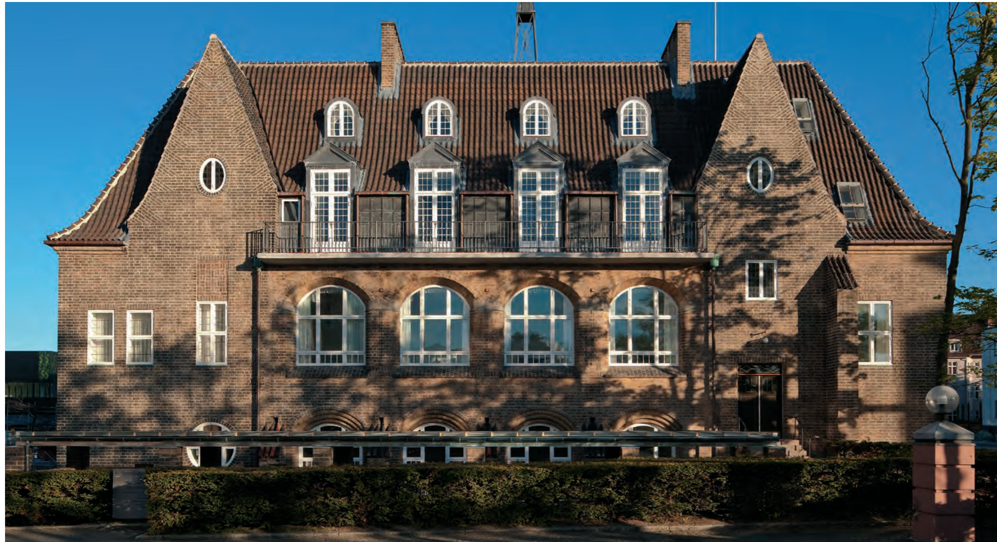
The Rosen House, the old administration building of former brewing company Tuborg built in 1913, was designed by the architect Anton Rosen as a Gesamtkunstwerk in the Skønvirke style, the Danish counterpart of Jugendstil and the British Arts and Crafts style.
