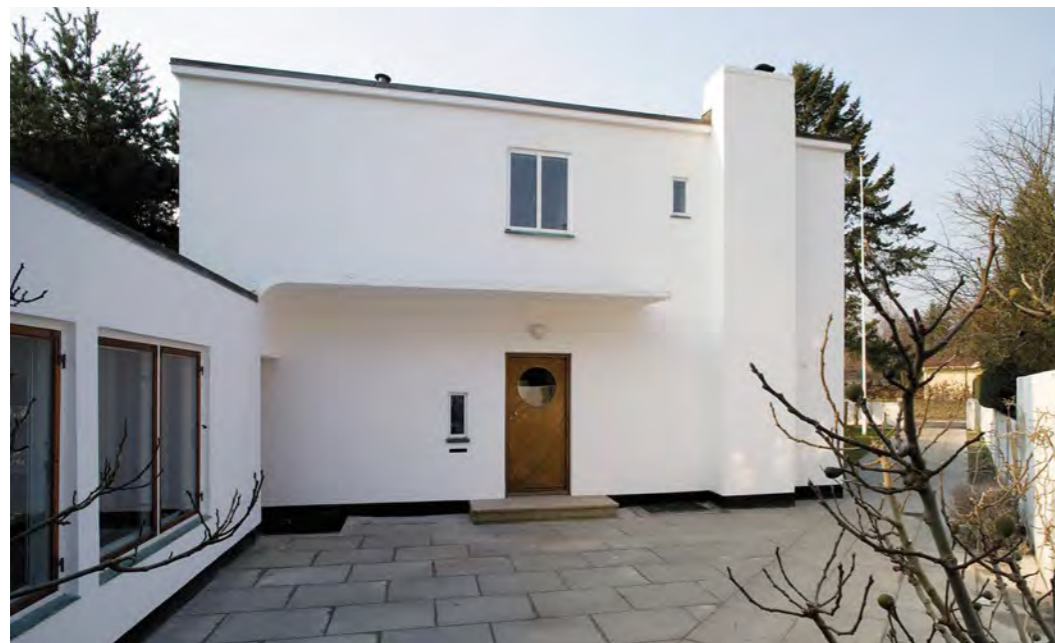
The drawing office wing, the house and the garden wall form a small triangular courtyard where you can quietly sit undisturbed.
