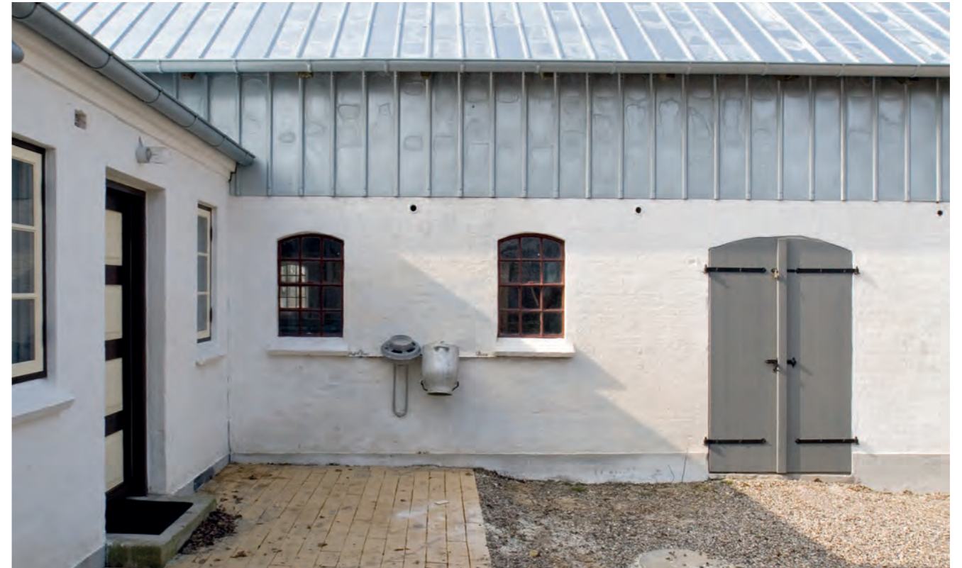
The restoration focused on enhancing the buildings' original qualities, so that the smallholding can speak to us today about the living standards, building practices and materials of yesterday.
